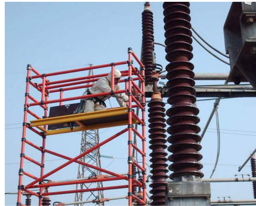
Work on isolators on high scaffold
