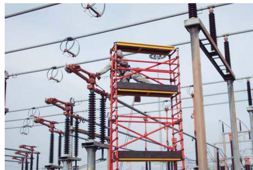
Work on isolators in a transformer station
