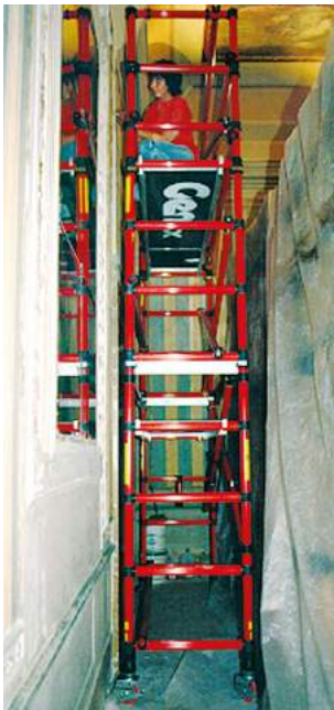
Custom-made scaffold for very narrow corridor
