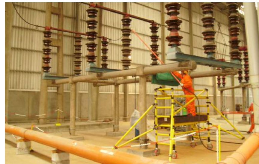
Work on isolators on low scaffold
